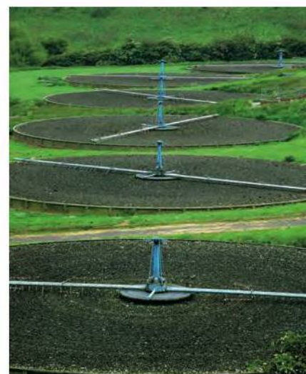
This is a trickling filter system at a sewage plant in Yorkshire, England. Have you visited the waste treatment plant in your community?
